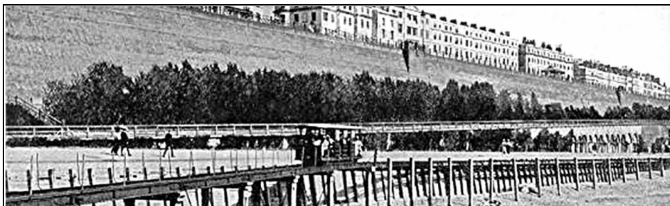
The viaduct east of Banjo Groyne from an undated postcard. Cars could be drenched by waves at high tide, indeed watching this seems to have been a source of entertainment. Sea defences have now allowed the beach here to build up almost to rail level affording the railway much better protection. Picture: Postcards of the Past (see back cover)
