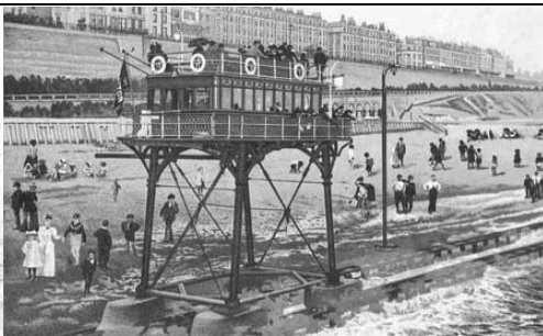
Left: Pioneer at the Rottingdean Pier which also housed the powerplant for the line. Rudyard Kipling rented a holiday home near Rottingdean and would fish from here when the railway was not in service. Right: Pioneer running at low tide. Pictures: Wikipedia under the Creative Commons licence.
